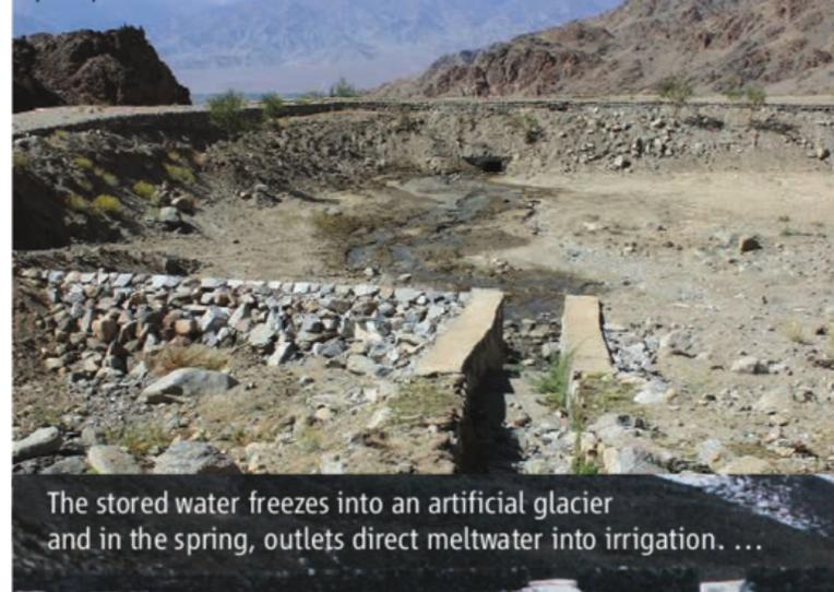
The stored water freezes into an artificial glacier and in the spring, outlets direct meltwater into irrigation. ...
