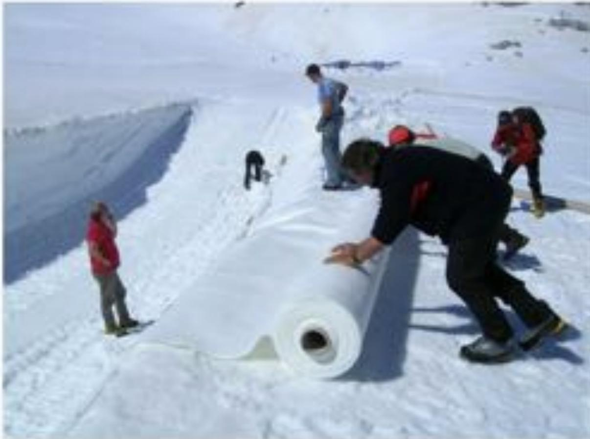
finally broke out the summer and the glacier Presena defends protecting under the "blanket" of geotextile fabrics expertly stretched by the workers of the company Carousel, which will prevent the sun's rays to penetrate and dissolve the precious snow. The hedging of the glacier started last week and have had to contend with a bizarre forecast that between Monday and Tuesday brought about 30 cm of fresh snow on the mountain.
